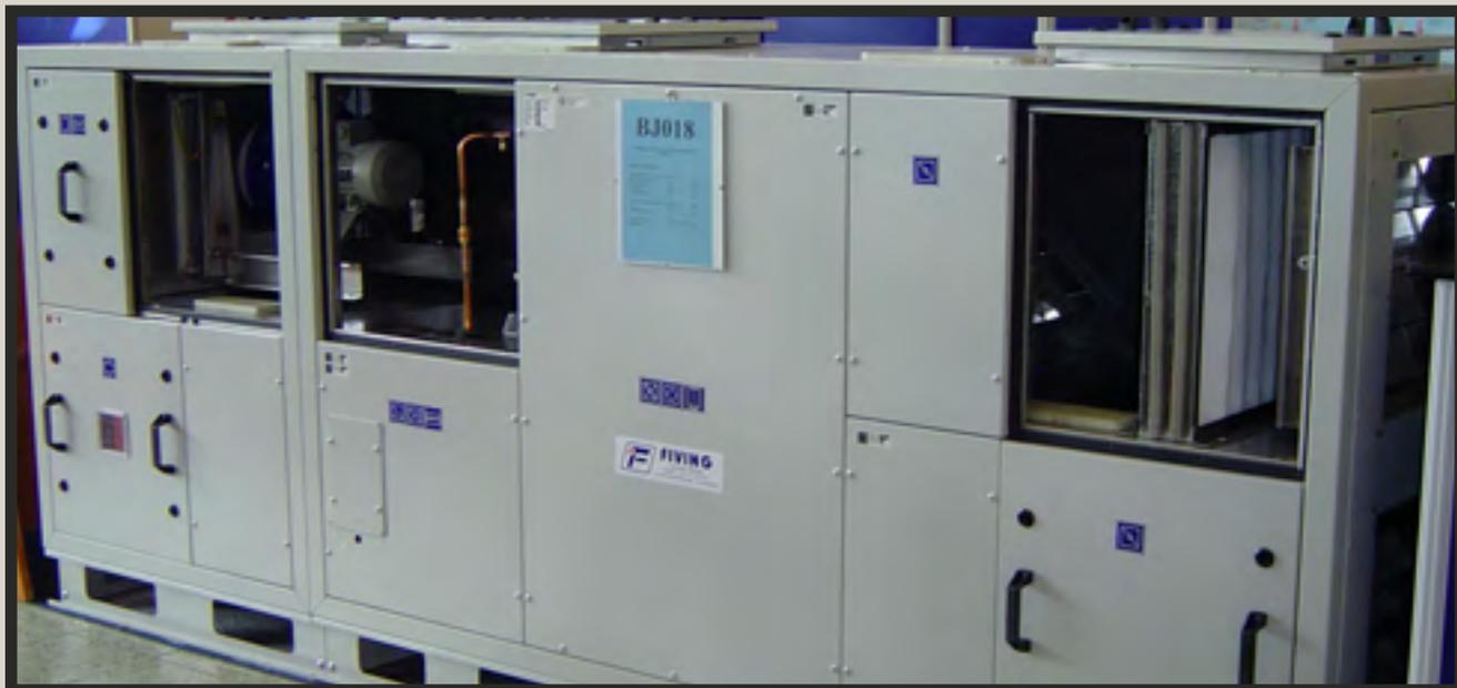
Air handling unit BJ is manufactured in 3 designs: outdoor, indoor, and hygienic. The size of the unit is chosen by the customer according to the requested parameters. All BJ device units can be equipped with a heat pump which uses heat from the surrounding air. The operation of such a device can save a considerable amount of energy, therefore, also funds spent on heating objects.
